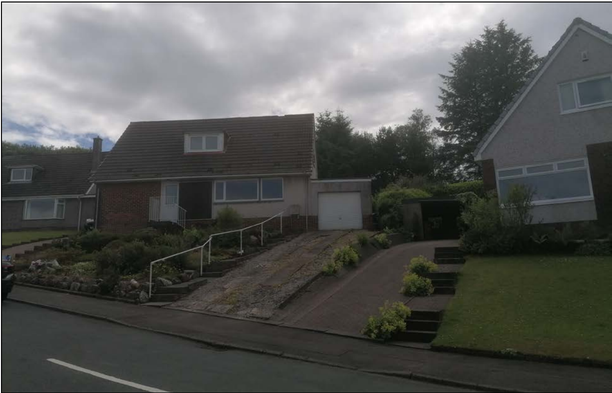
View of the front of the property from Rosemount Place.
